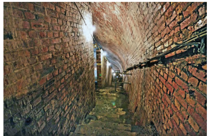
North side stairs with upper level access to shelter section 3 visible
